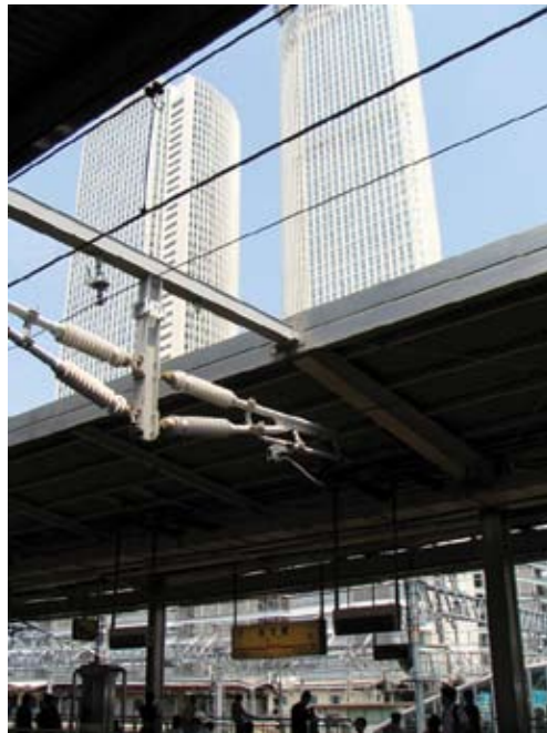
High-speed rail stations have the potential to attract many forms of development, including offices, hotels, retail stores and entertainment venues. Above, the 50-story-plus JR Towers rise above Tokyo's Nagoya rail station. Credit: Steve Boland, Nelson/Nygaard Consulting Associates
