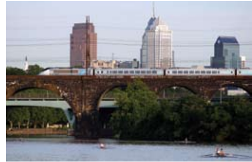
Despite operating over aging infrastructure, Amtrak’s Acela Express near-high-speed rail service on the East Coast competes effectively with air travel. Credit: Kyle Gradinger
