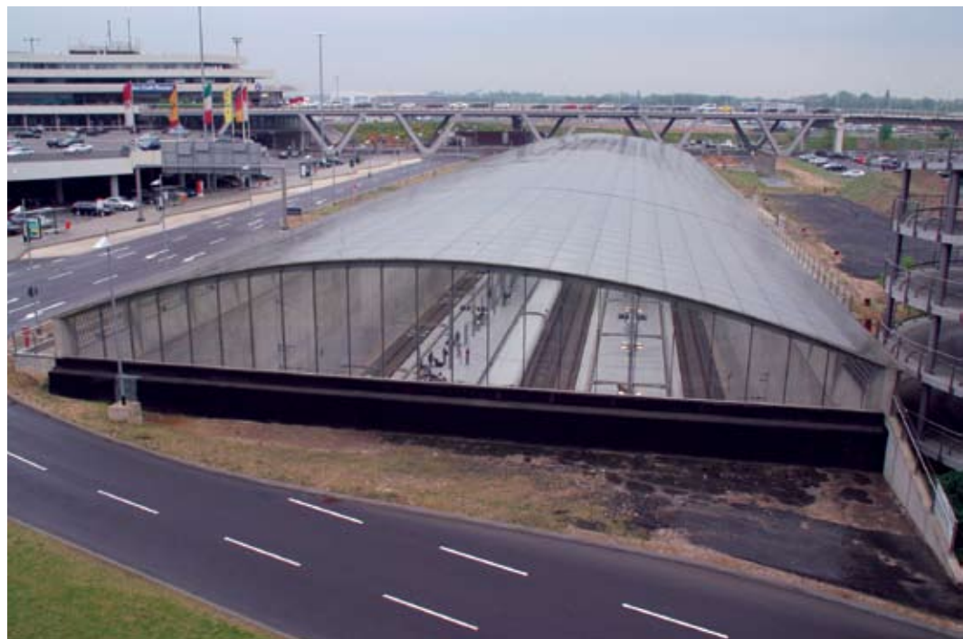
Locating high-speed rail stations at airports can enable airlines to replace energy-inefficient connecting flights that clog up gate space. The Intercity Express rail station at the airport in Cologne, Germany (above), provides direct access to the high-speed rail network connecting Germany and other nations in northern Europe, enabling travelers flying into Cologne to reach their final destination elsewhere in the country more quickly and conveniently. Credit: Gregorius Mundus
